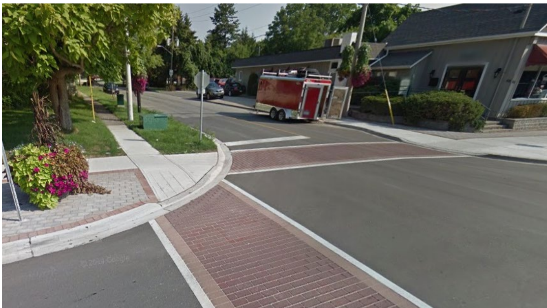
Figure 29: Example of Coloured Impressed Asphalt
