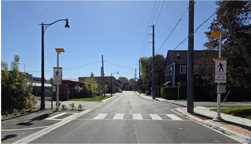
Figure 23: Pedestrian Crossing on Edward Street in the Town
