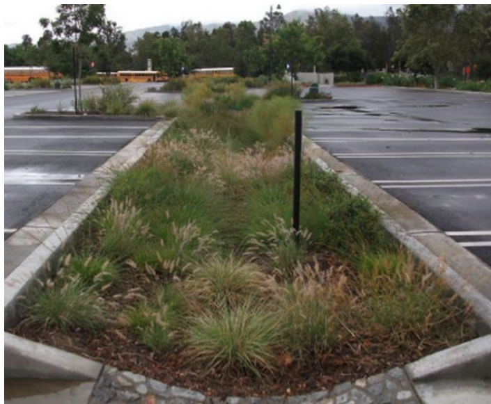
Figure 46: Example of a Vegetated Bioswale
