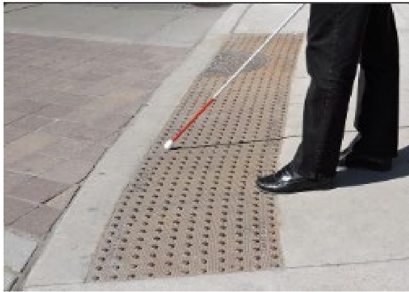
Figure 26: Tactile Plate (with drop curb)
