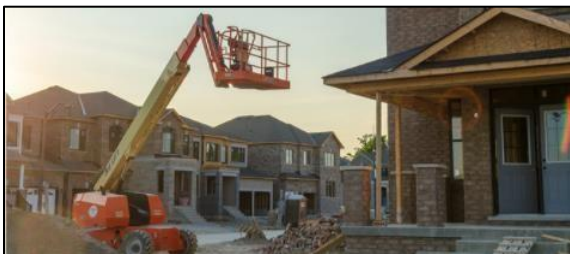
Figure 6: Construction Activity in the Town of Whitchurch-Stouffville
