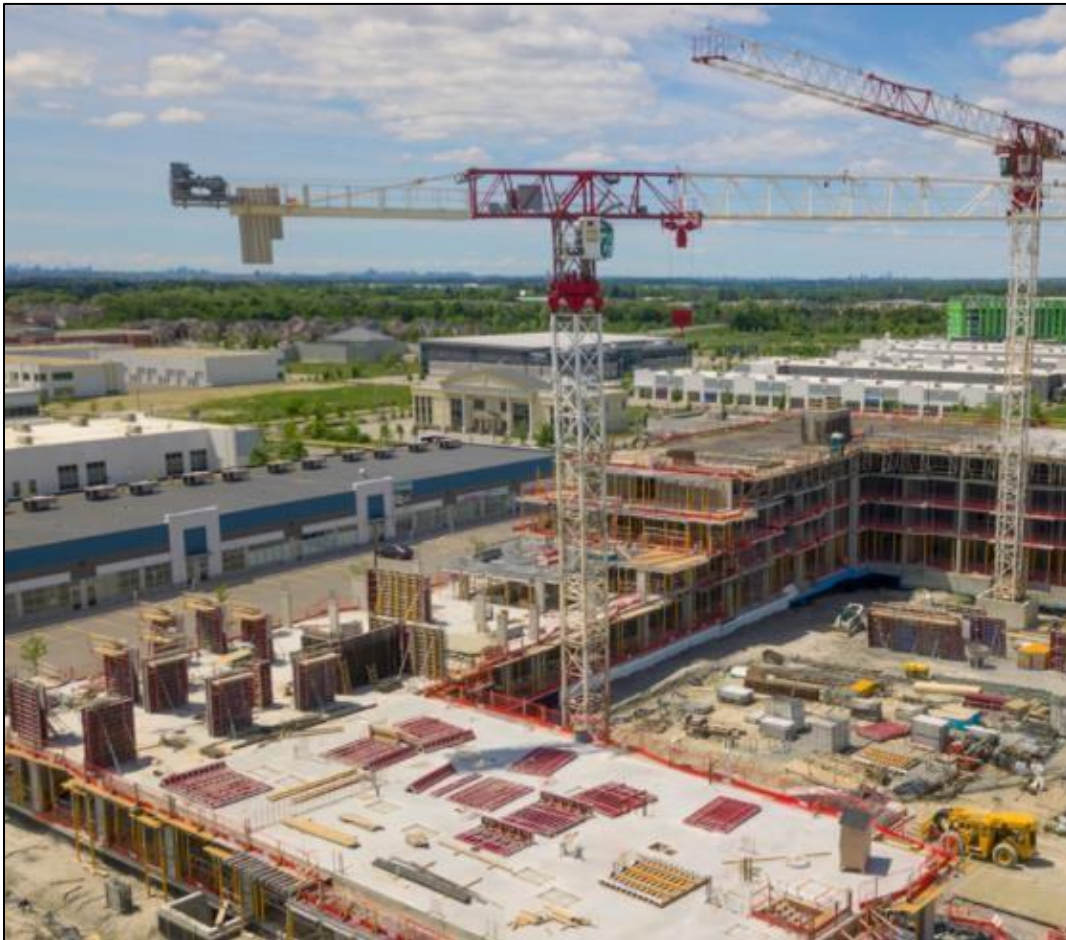
Figure 5: Construction Activity in the Town of Whitchurch-Stouffville
