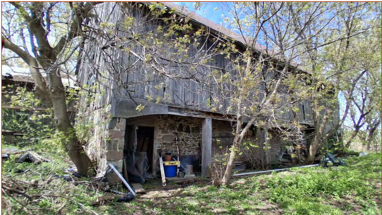
Photo 15. View of the south elevation of the barn with access to the ground level.
