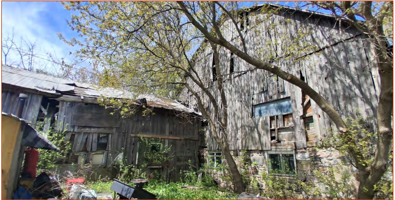
Photo 13. View of the west elevation of the barn and the connection to the barn addition.
