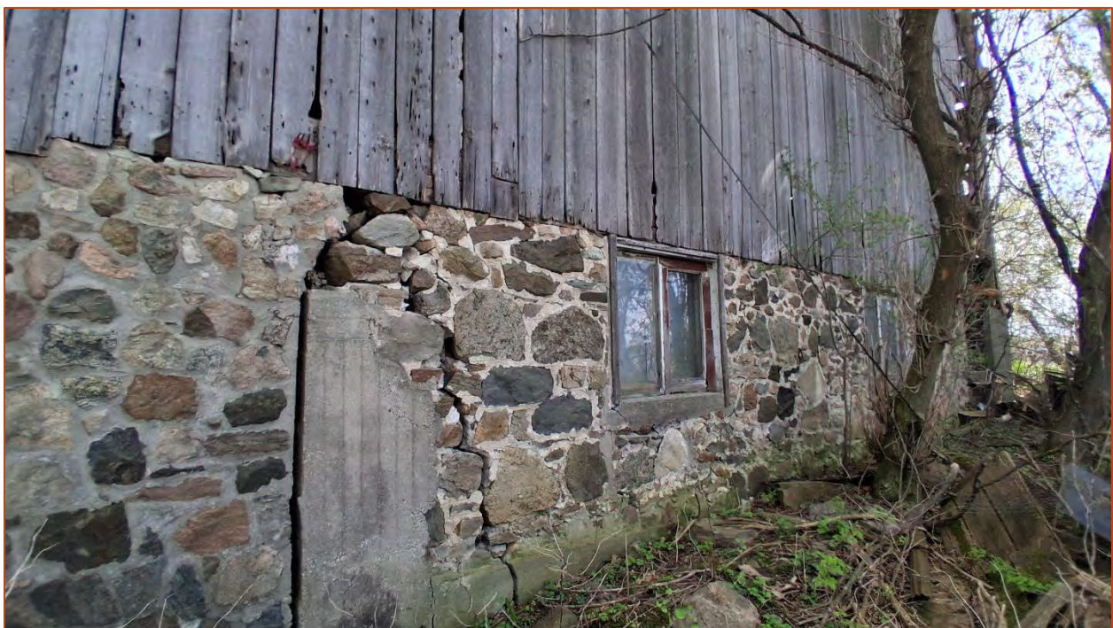
Photo 16. Detailed view of the east elevation foundation.
