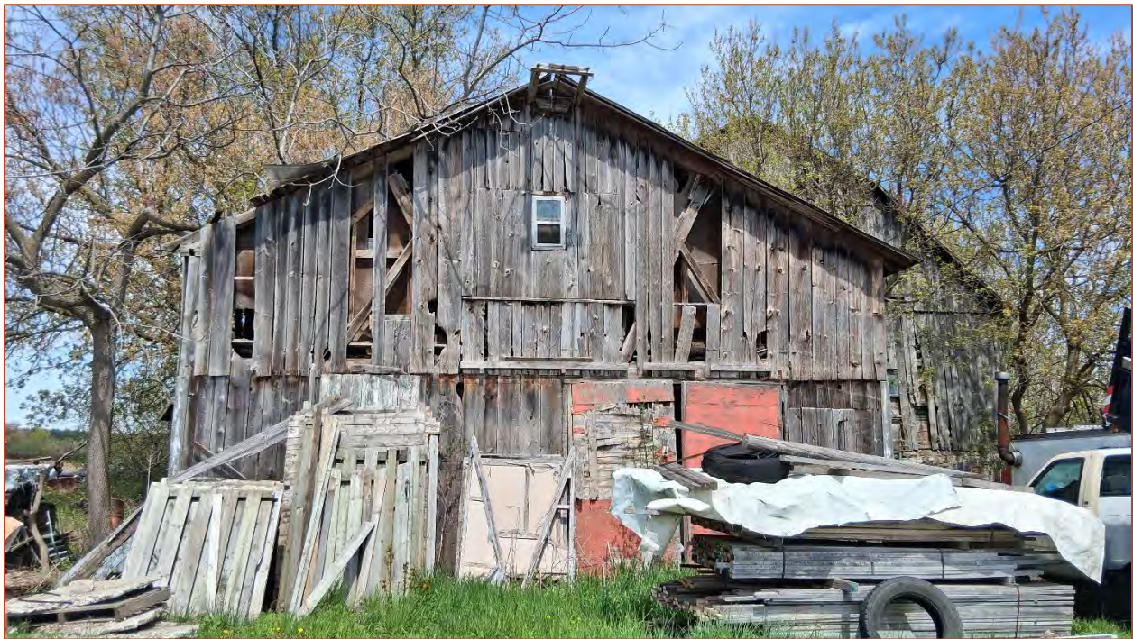
Photo 24. View of the west elevation of the barn addition.
