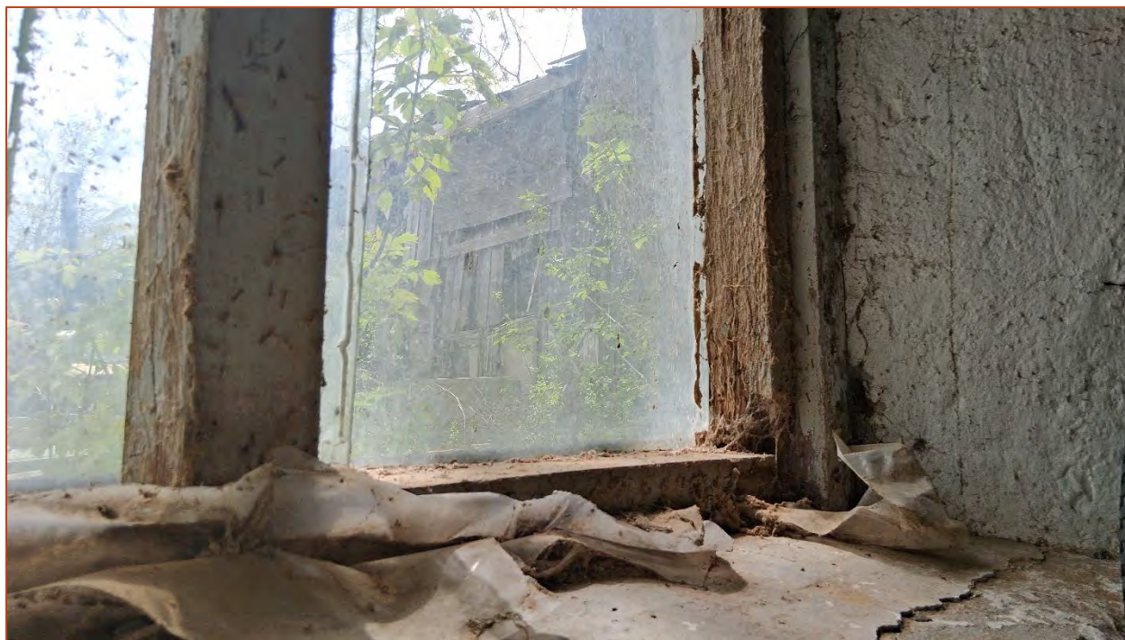
Photo 18. Detailed view of a window frame.
