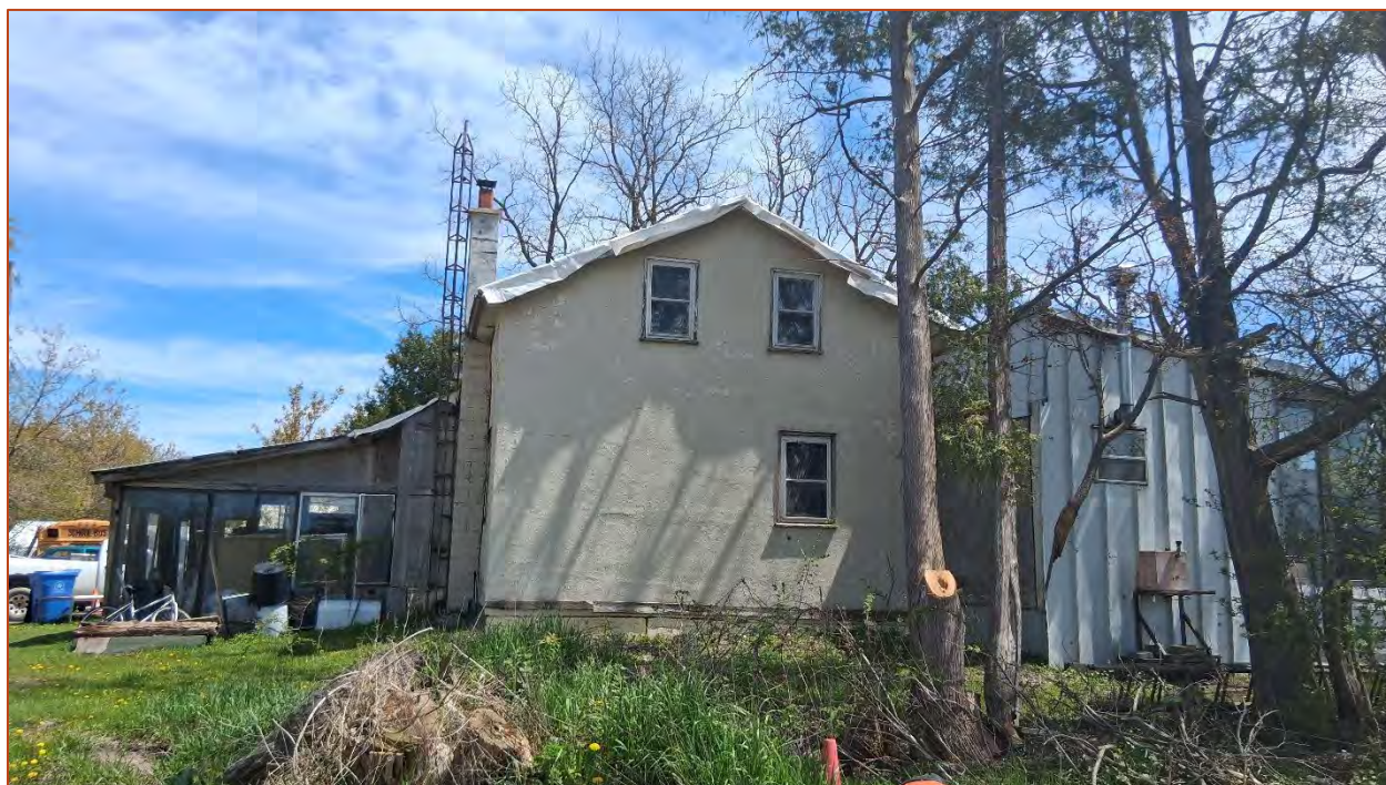
Photo 9. View of the north elevation.
