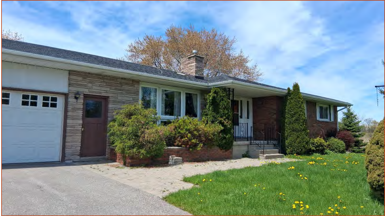
Photo 31. View of the façade (east elevation).
