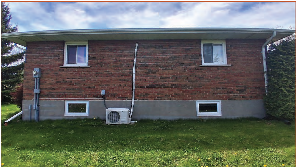
Photo 32. View of the north elevation.
