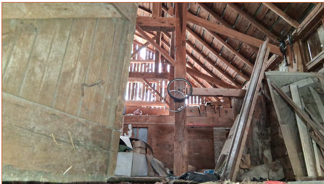
Photo 23. Interior view of the second-floor hayloft.
