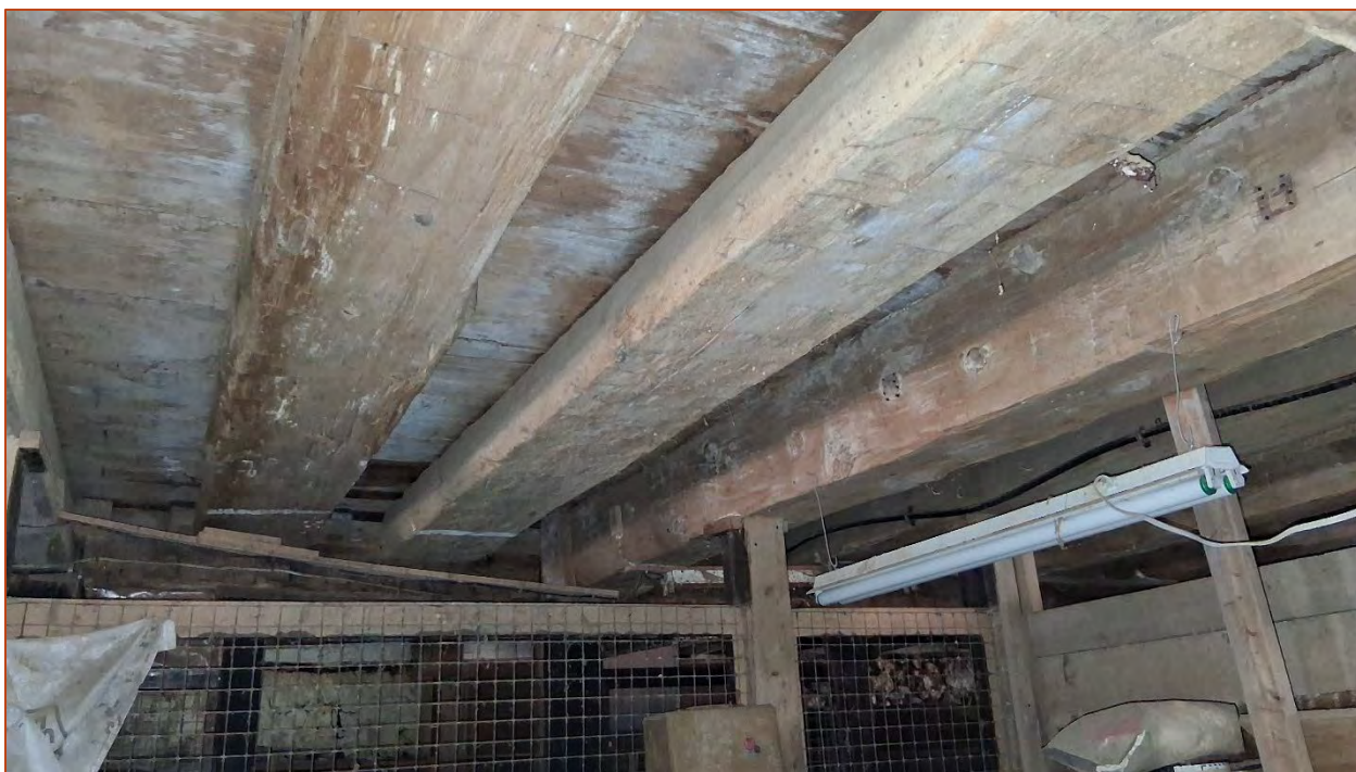
Photo 21. Interior view of large axe-hewn timber beams with a noticeable gap from the ceiling.
