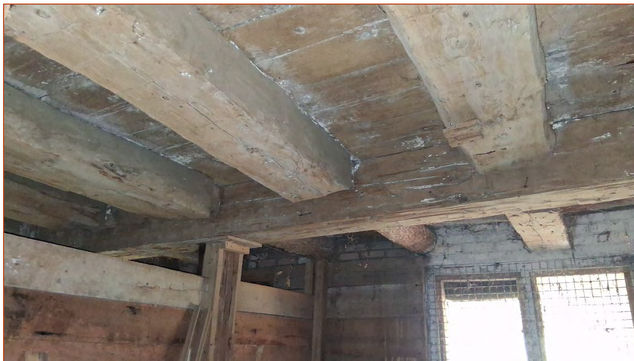
Photo 22. Interior view of large axe-hewn timber beams and brick headers.
