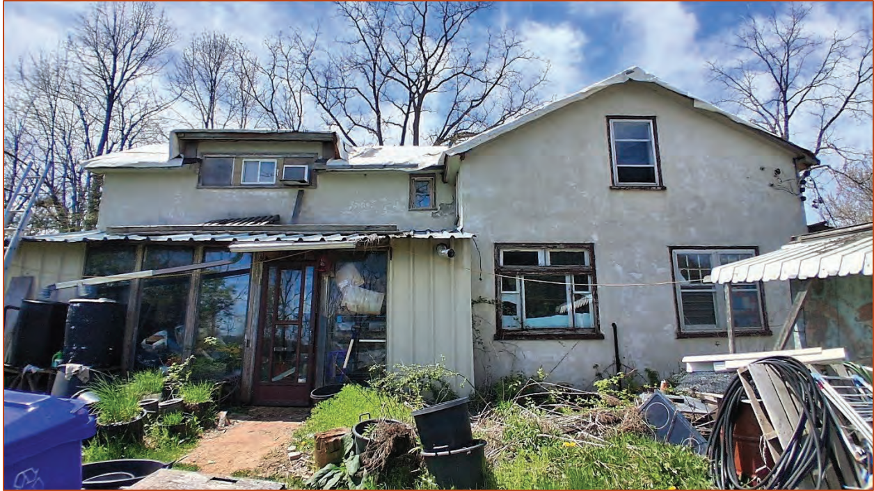
Photo 12. View of the south elevation.
