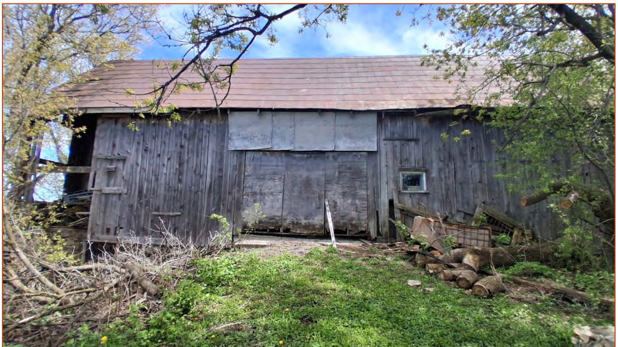
Photo 14. View of the north elevation of the barn with the access ramp to the second-floor hayloft.
