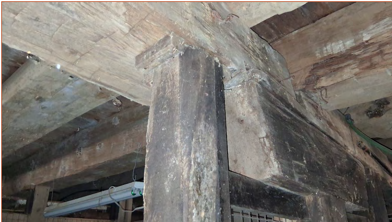
Photo 20. Interior view of large axe-hewn timber posts and beams.
