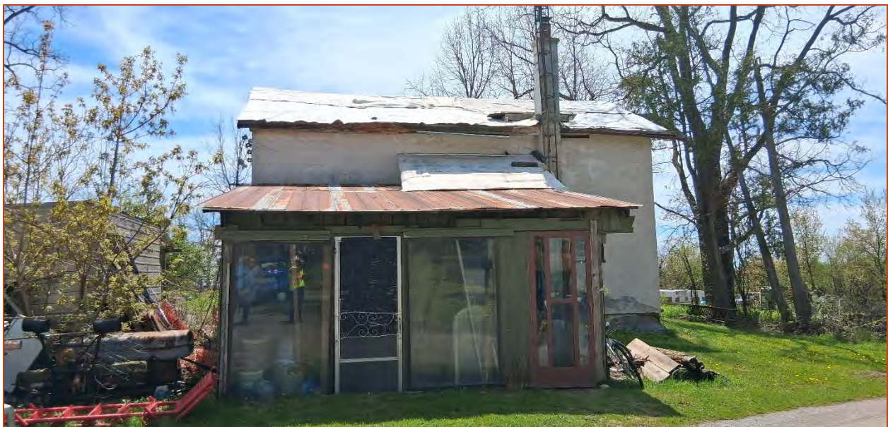
Photo 7. View of the façade (east elevation).
