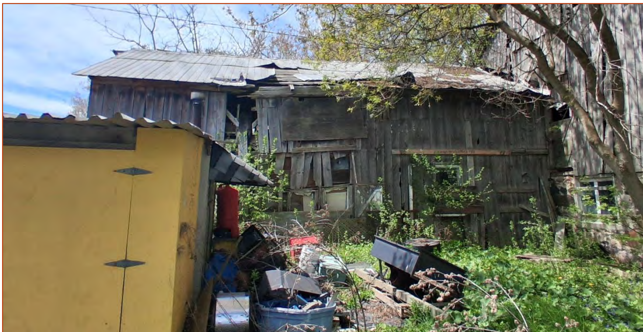
Photo 26. View of the south elevation of the barn addition.
