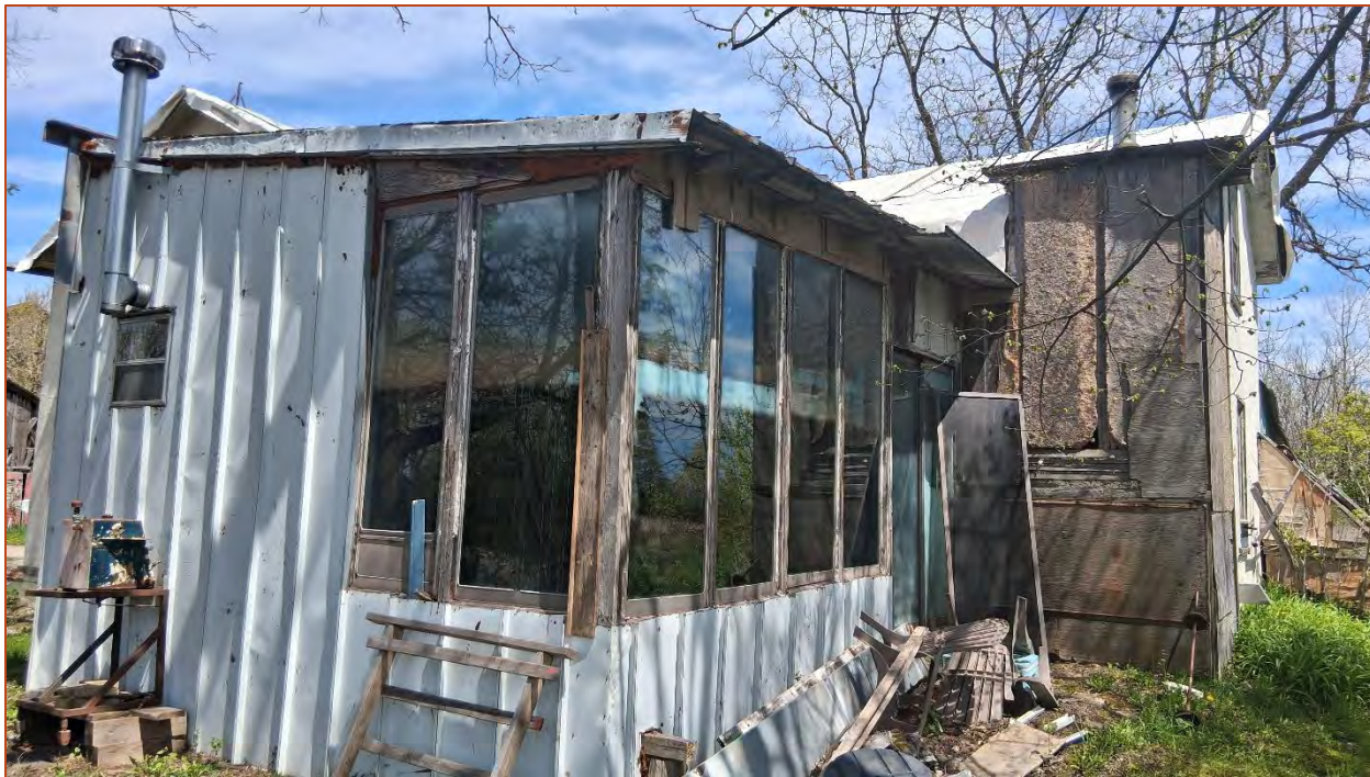
Photo 10. View of the north elevation including the lean-to additions.
