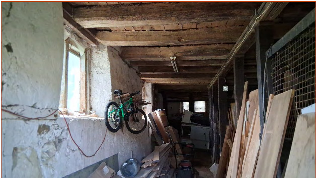
Photo 17. Interior view of the barn showing the limewashed fieldstone foundation wall at left.
