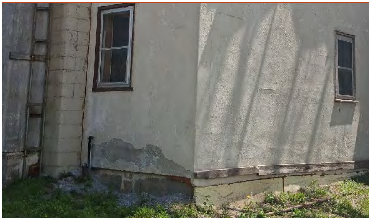
Photo 8. View of the fieldstone foundation.
