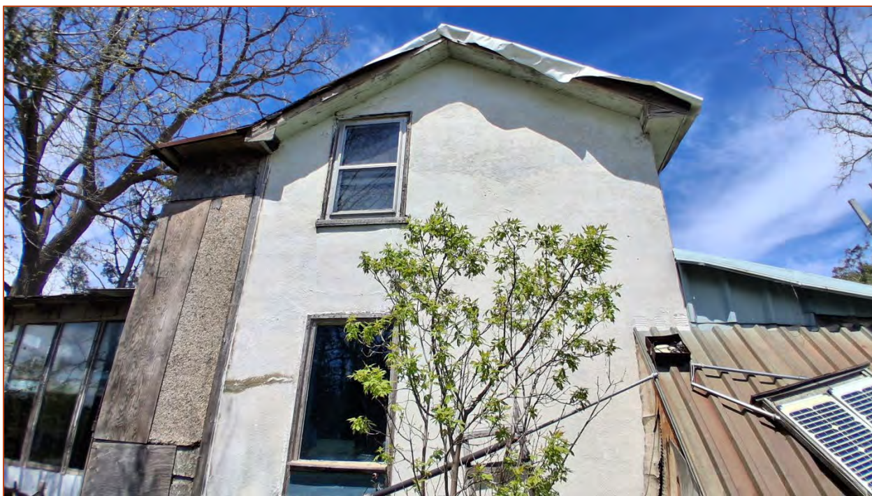
Photo 11. View of the west elevation.
