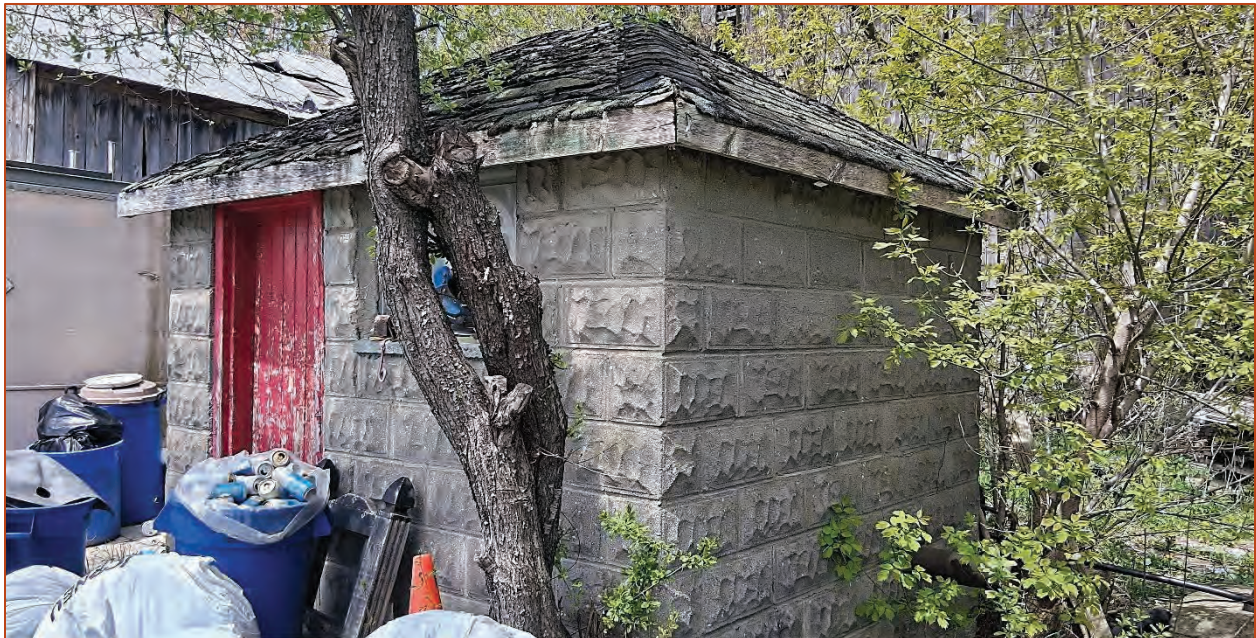
Photo 27. View of the pumphouse building.
