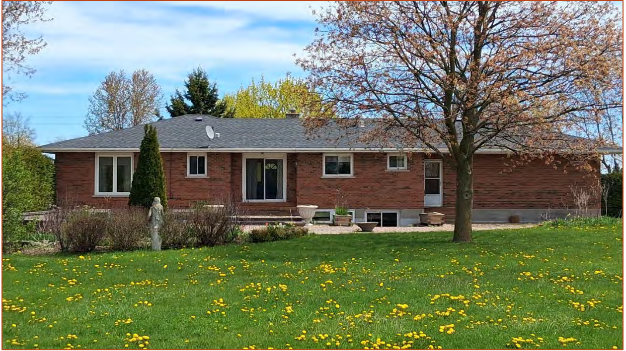
Photo 33. View of the west elevation.
