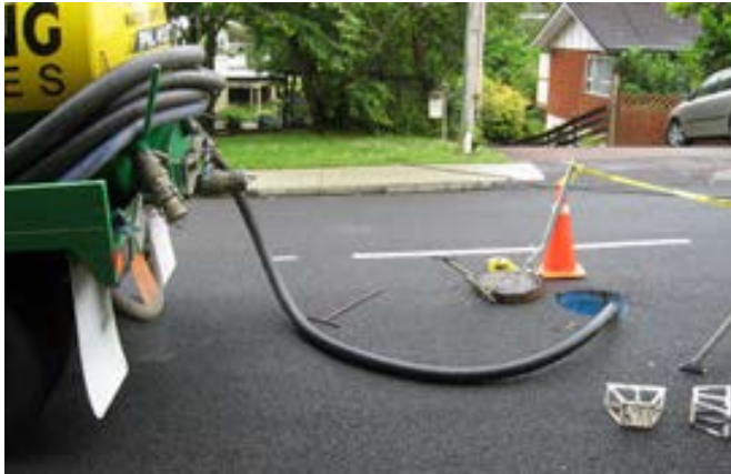
Figure 2: Sediment is removed from the sump with a vactor hose. Confined space entry is not required for this step.
