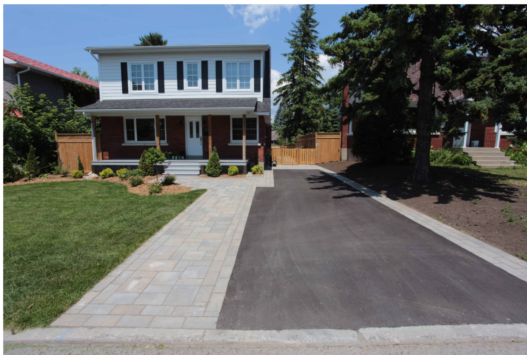
Example of a Driveway Expansion
