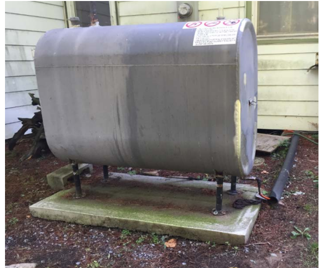
Photograph 4. View of the fuel oil tank on the east side of the older residence at 5584 Lakeshore Road. (September 2016)
