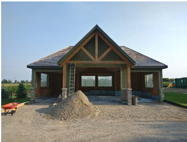
Photograph 15. View of garage under construction at 5584 Lakeshore Road. (August 2018)
