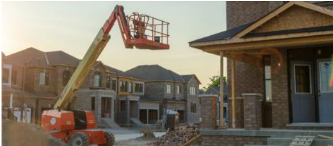
Figure 7: Construction Activity in the Town of Whitchurch-Stouffville
