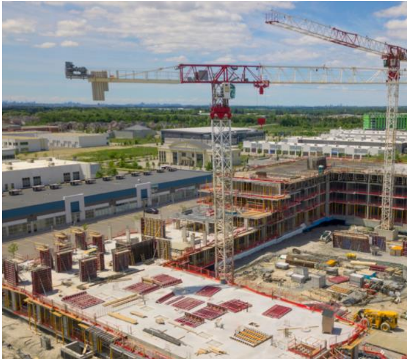
Figure 8: Construction Activity in the Town of Whitchurch-Stouffville
