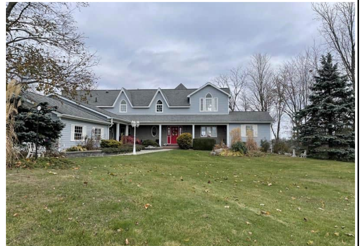
PHOTO 4: View of the residential dwelling located on the Phase One Property, facing northeast.
