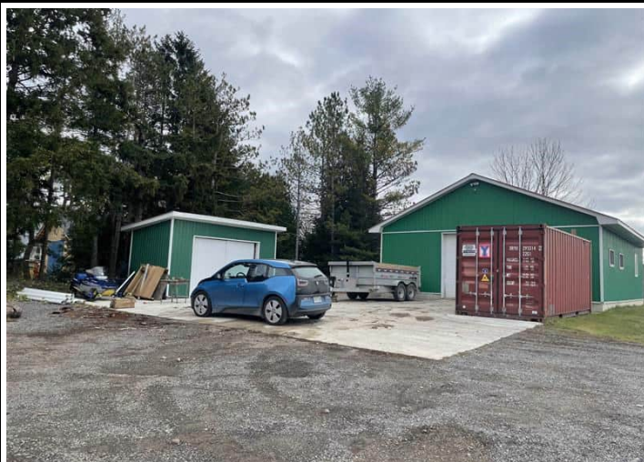
PHOTO 7: View of the large shed located at the Phase One Property, facing northeast.
