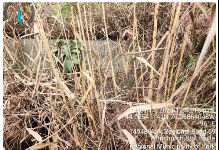
PHOTO 4: View of the head wall located on the southern portion of the Conveyance Lands, facing east.
