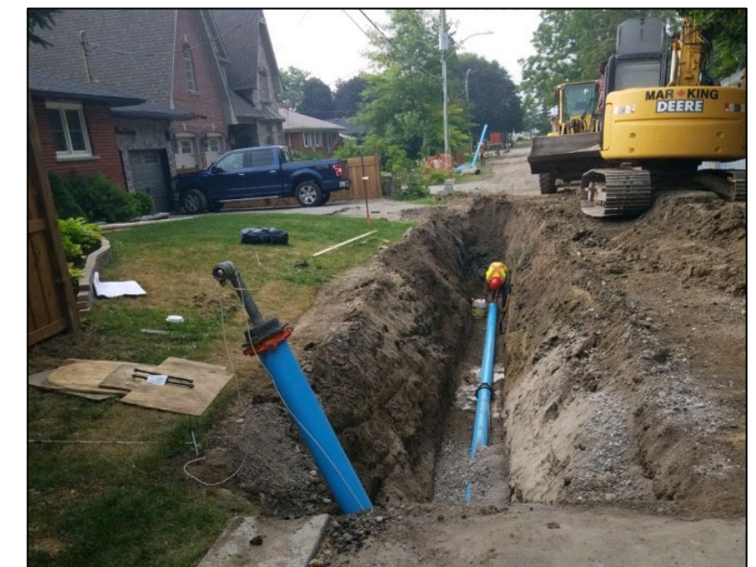
Watermain Installation on Burkholder Street
