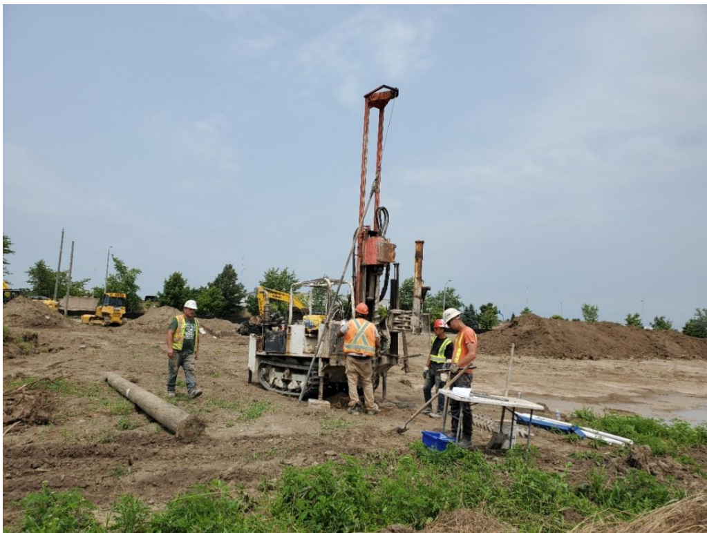
Photograph 3: Facing north on the southwest portion of the property showing borehole drilling during the Phase II investigation.
