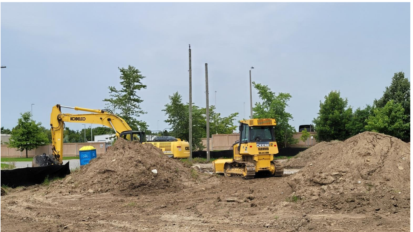
Photograph 2: Facing north on the west portion of the property showing construction equipment used for topsoil stripping.
