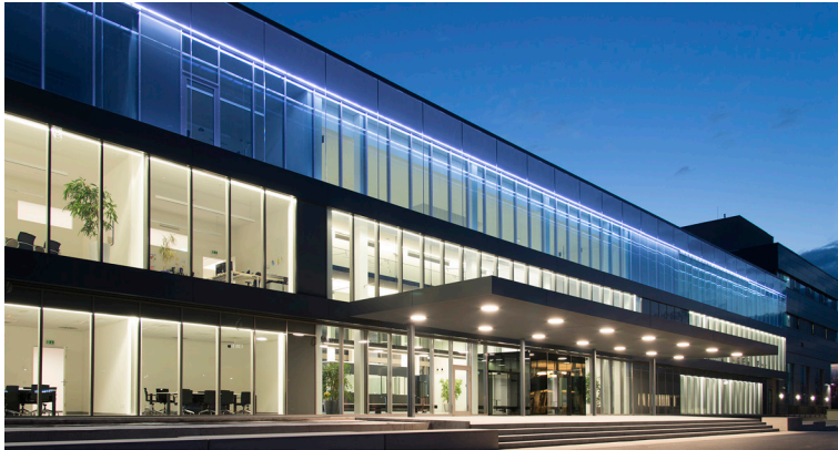
Office building that located at the street
