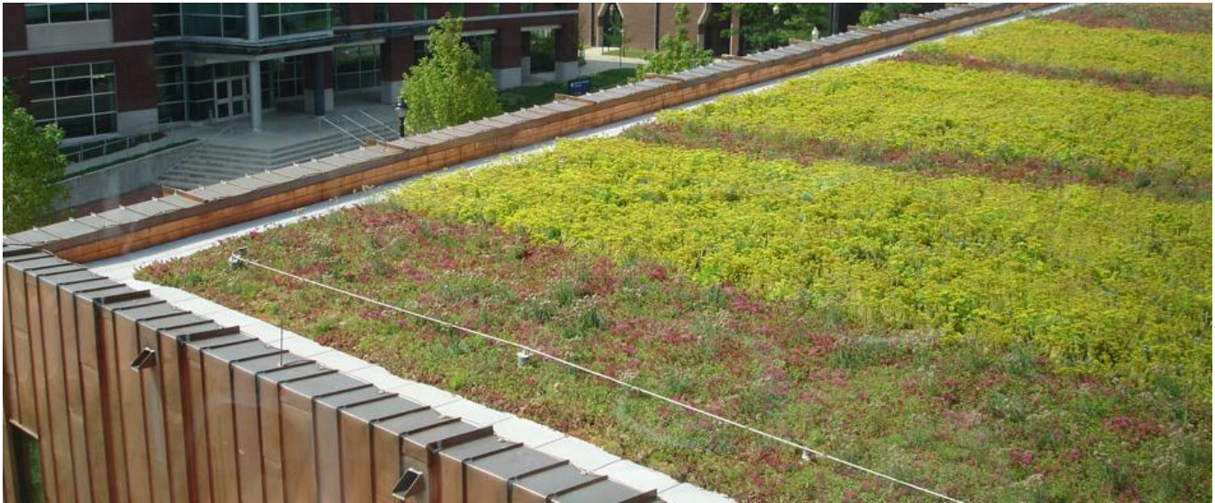
Figure 4-10: Green Roof Example
