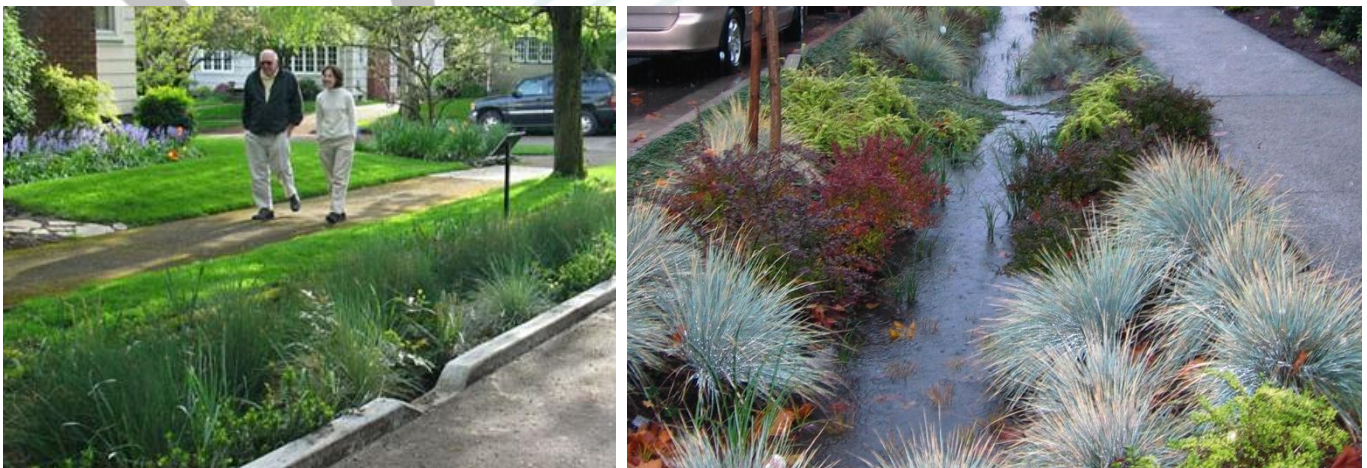
Figure 4-15: Bioswales in the Public Realm
