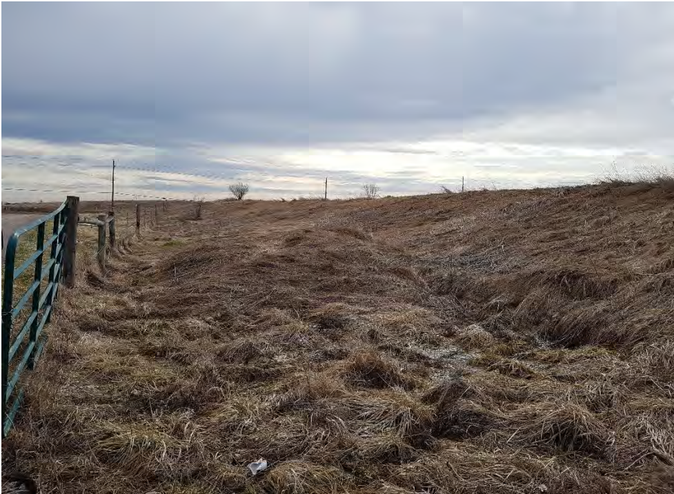
Image 3: Manufactured berm slope along northern fence line of property, view north-east.
