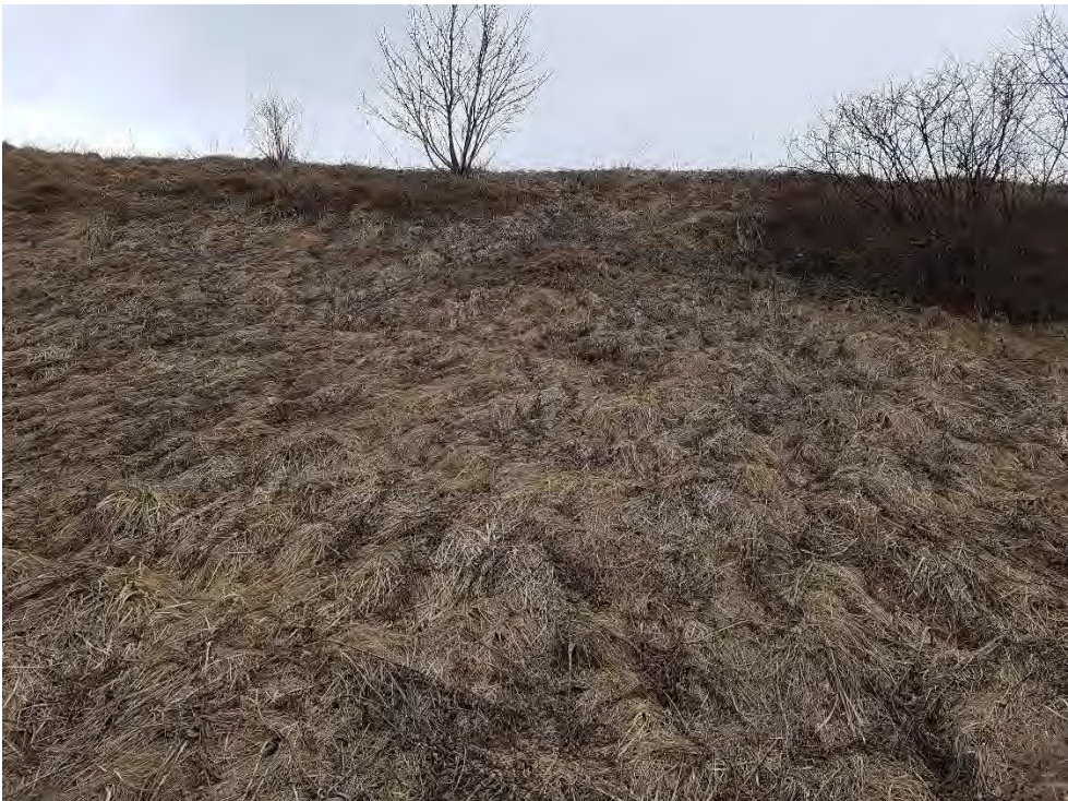
Image 10: View of steep slope from mid-point of manufactured berm, view south-southeast.
