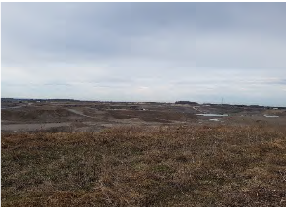
Image 6: View of open excavation from gravel road along berm, view southwest.
