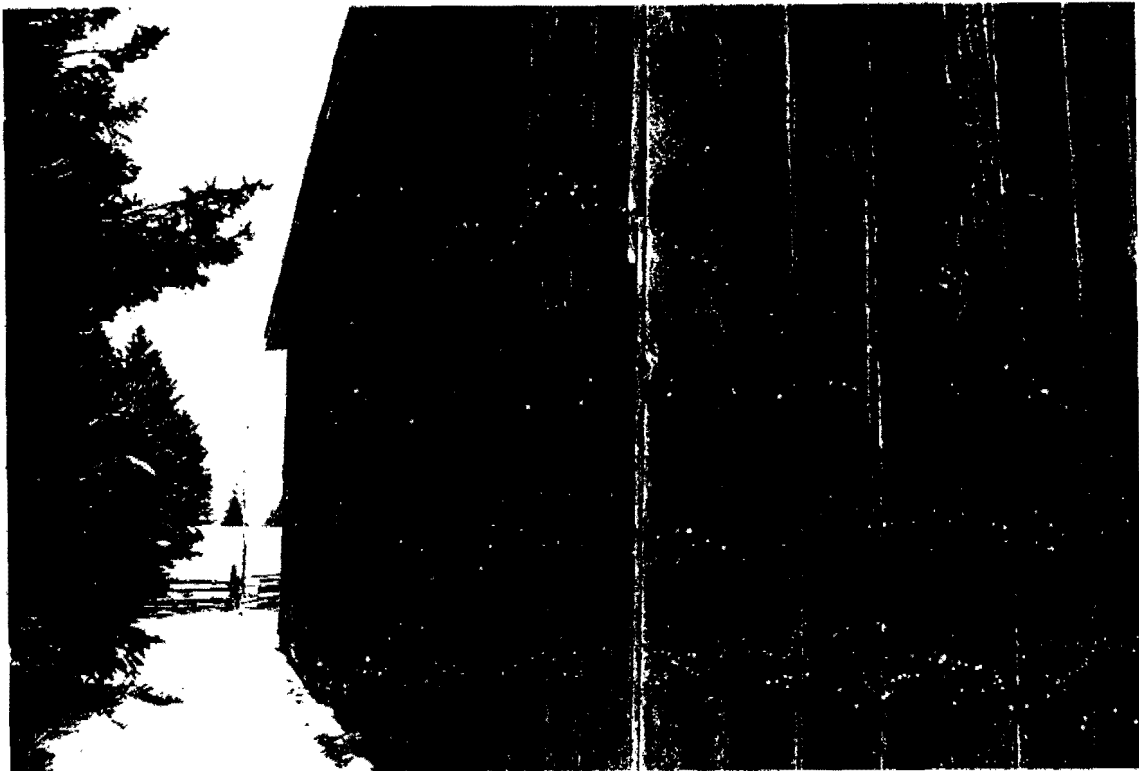
West Facade. Note decorative effect created by the overlap of vertical planks.
