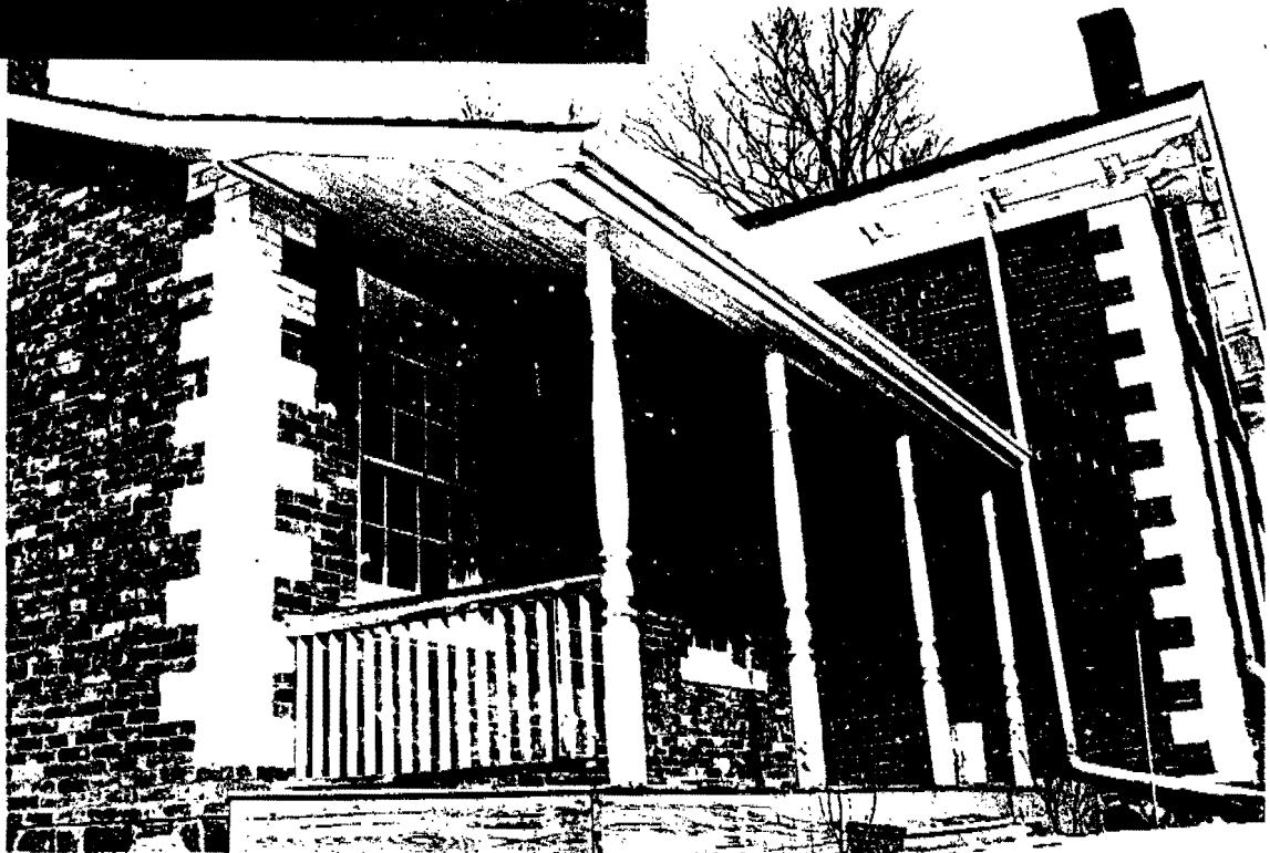
South verandah on kitchen tail
