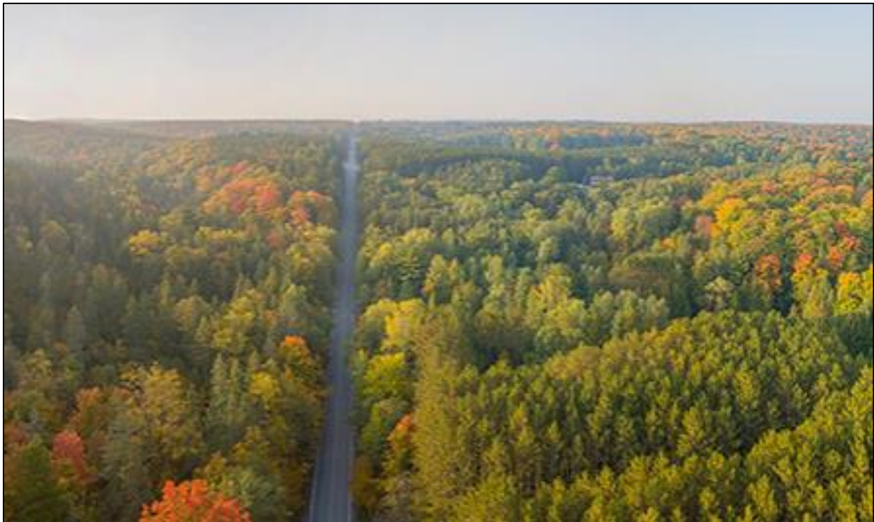
Figure 3: Town of Whitchurch-Stouffville Aerial View
