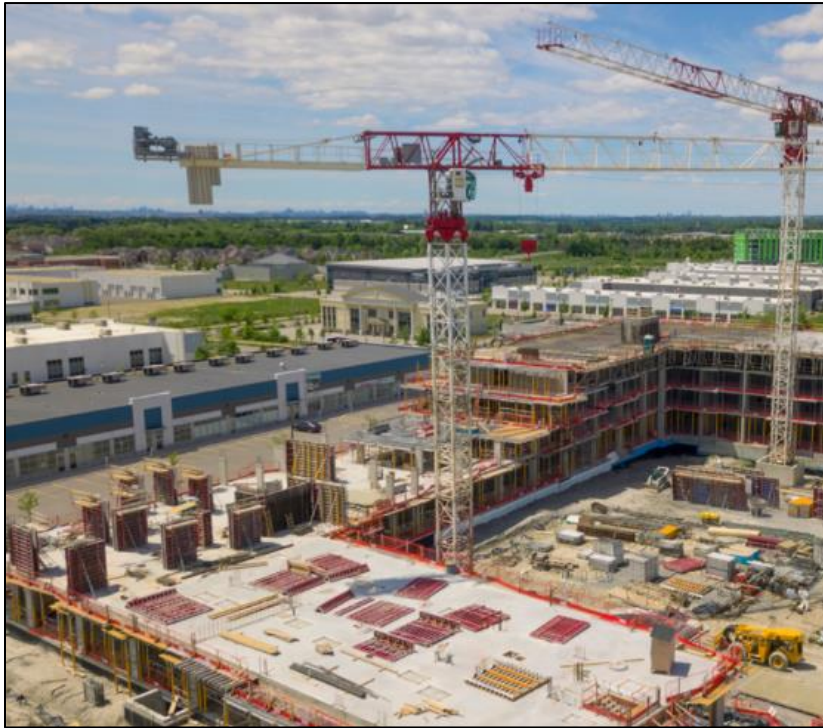
Figure 8: Construction Activity in the Town of Whitchurch-Stouffville
