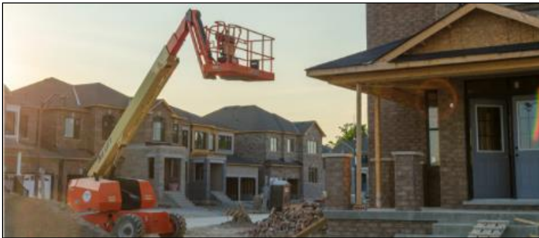
Figure 7: Construction Activity in the Town of Whitchurch-Stouffville
