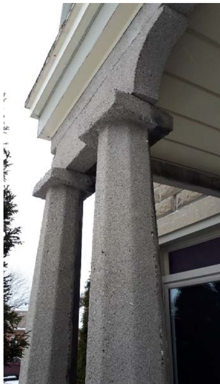
A closer view of concrete columns with a simple square capitals and entablature. Pre-war concrete porches are fairly rare features and likely the only ones existing in the municipality (Parsons, 2019).
