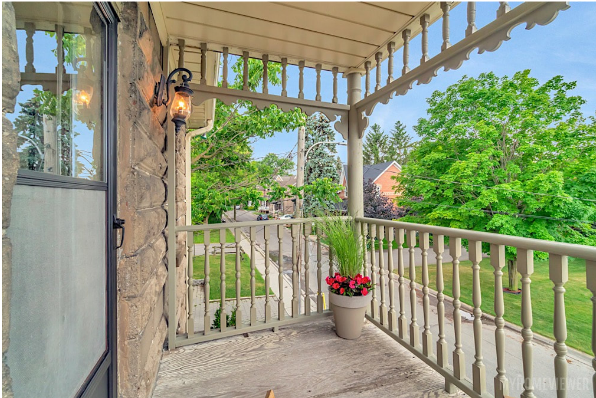
Showing the condition of the porch's upper balcony. The decorative wood trim and balustrade accents, although not original features, provide a complimentary accent to the standardized rusticated concrete cladding (Trentadue Torres Group, 2019).
