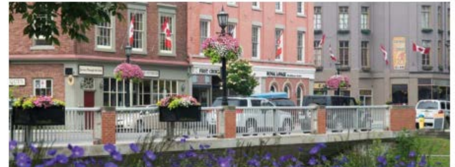
Bridge over Ganaraska River in Port Hope.
