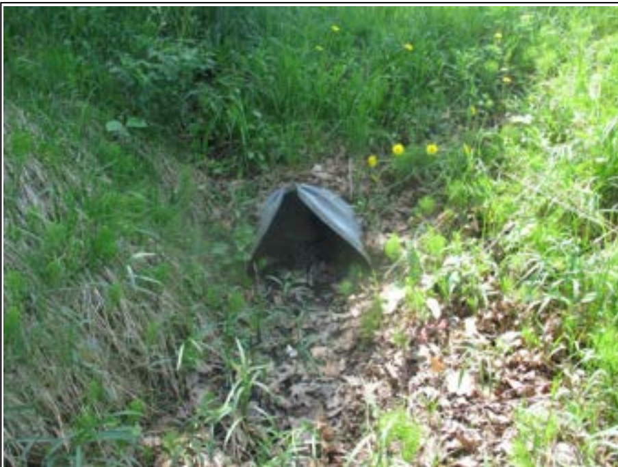
CSP beneath Edward St., E outlet – May 30, 2018
