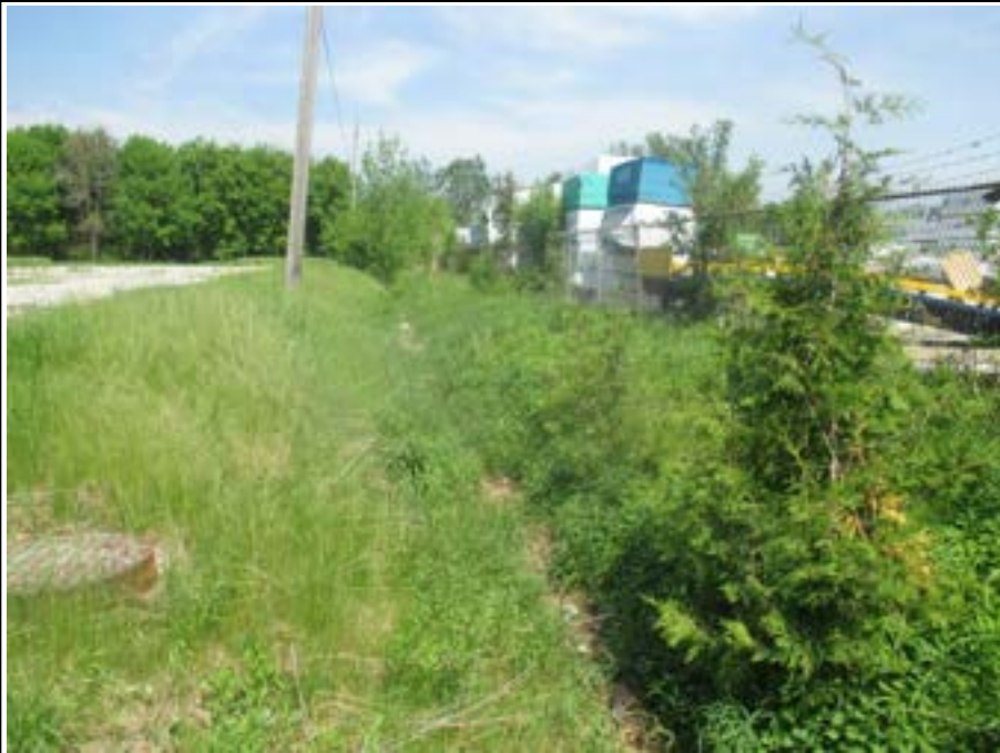
Drainage channel from study area limit, facing E – May 30, 2018
