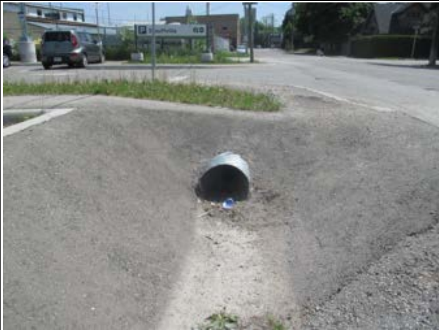
Municipal drainage ditch, E side Edward St. – May 30, 2018
