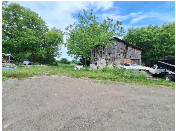
Image 14: Structure within project area, facing north.
