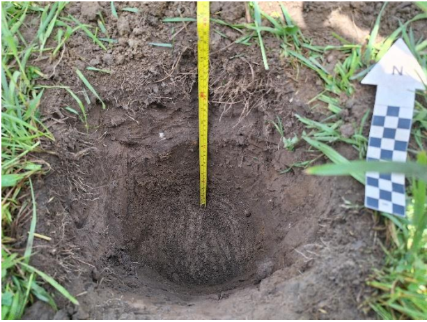
Image 19: Typical test pit.
