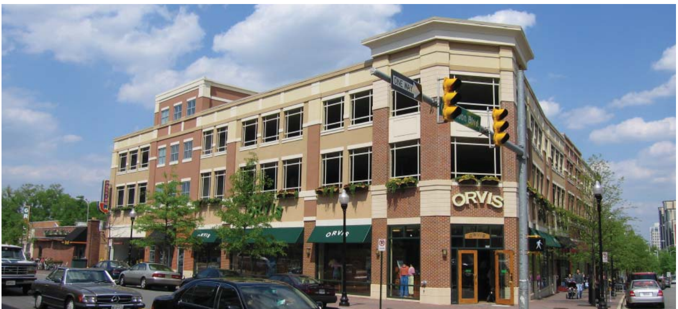
Structured parking garages should be carefully designed to ensure they are compatible with the scale and massing of adjacent buildings.
