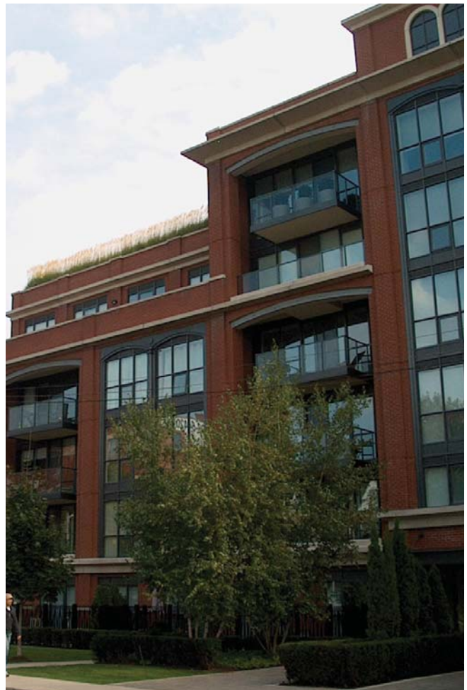
Buildings should step-down to transition towards adjacent low-rise neighbourhoods. Green roofs are encouraged to provide intriguing views for residents, and to enhance the public perception at street level.
