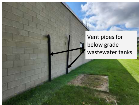
Photo 6: View of a the two (2) vent pipes for below grade wastewater tank located exterior adjacent to the west wall of the Site building.
