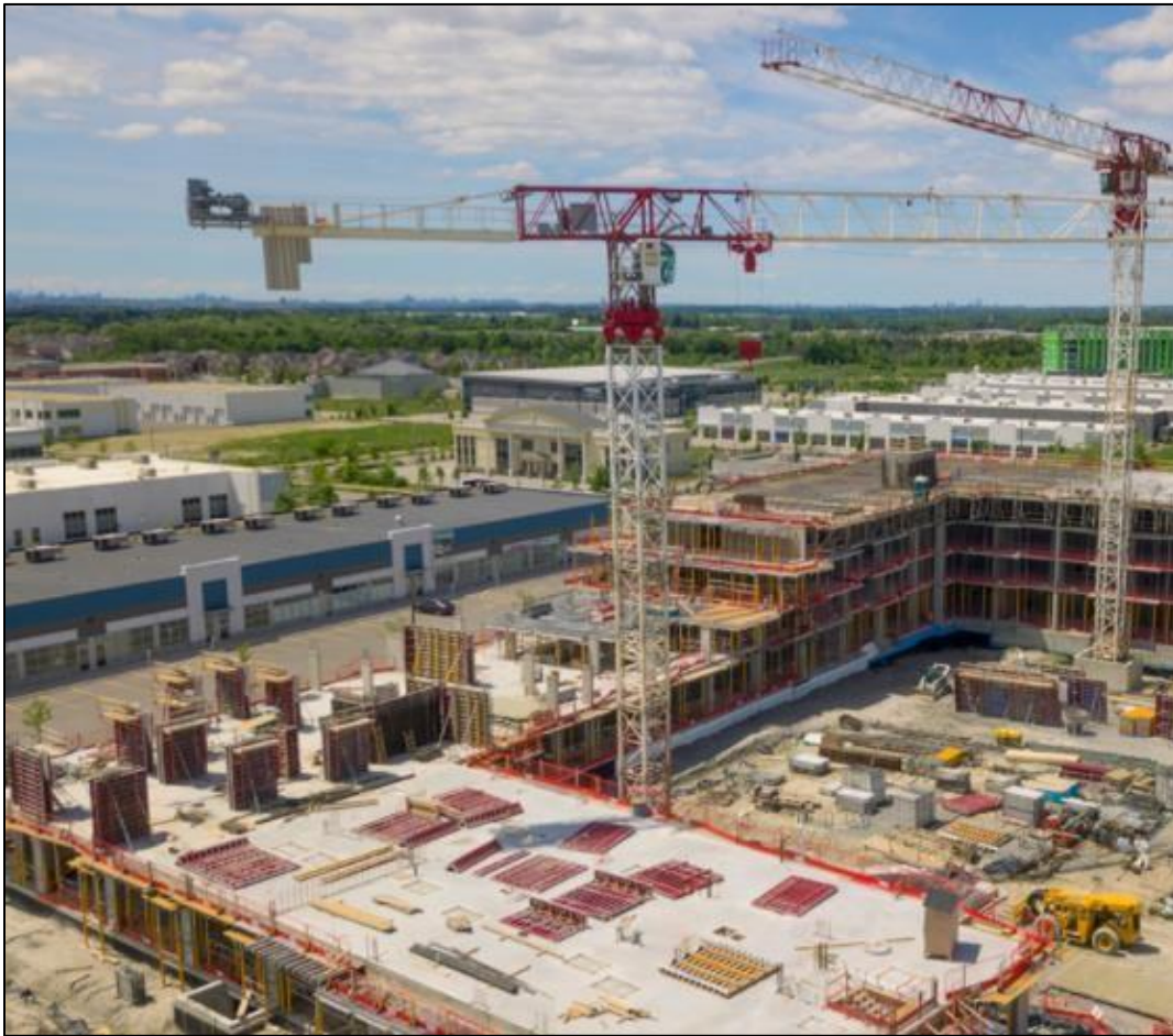
Figure 5: Construction Activity in the Town of Whitchurch-Stouffville
