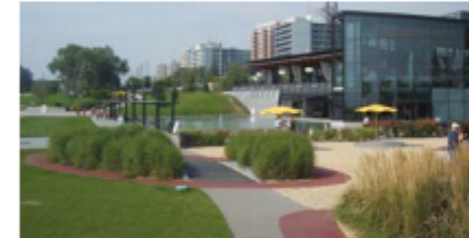
Market Commons multi-residential project in Burlington.
