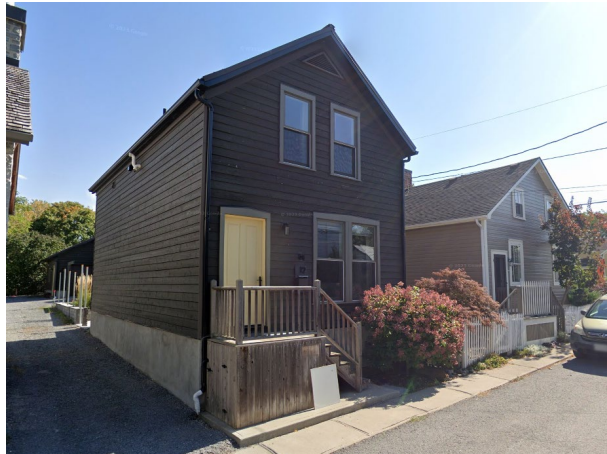
Photo credit: Google StreetView
